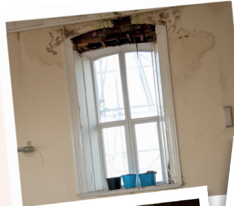
Windows before the work began
