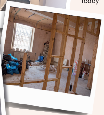
Ground floor as work began
